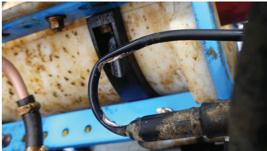
Figure 3-39 – Recovered NSIF OPTAA pump cable with jacket tears and loose locking sleeve
