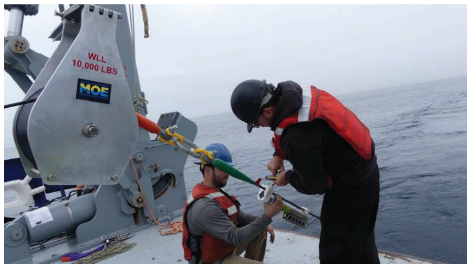
Figure 3-6 – Installing the 1500 m CTDMO on the GI01SUMO-00006 mooring
